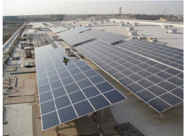
Fig. 3 A 667 kW PV array at the rooftop of QNCC [12].
